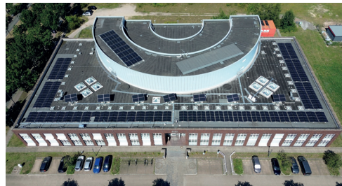
Left: High-level overview of the components and interrelationships of the IdEaL Model Factory | Above: Drone footage of BIBA with solar installations as part of the energy flexibility concept, Sources: BIBA GmbH
