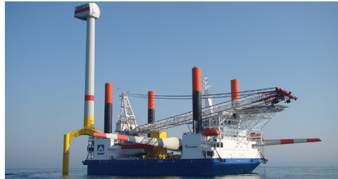
Left: Installation of a Preassembled Rotor Star, Photo: Hochtief Above: Loading of Rotor Blades, Photo: Servnion
