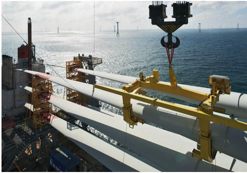
Left: Installation of a Preassembled Rotor Star, Photo: Hochtief Above: Loading of Rotor Blades, Photo: Servnion
